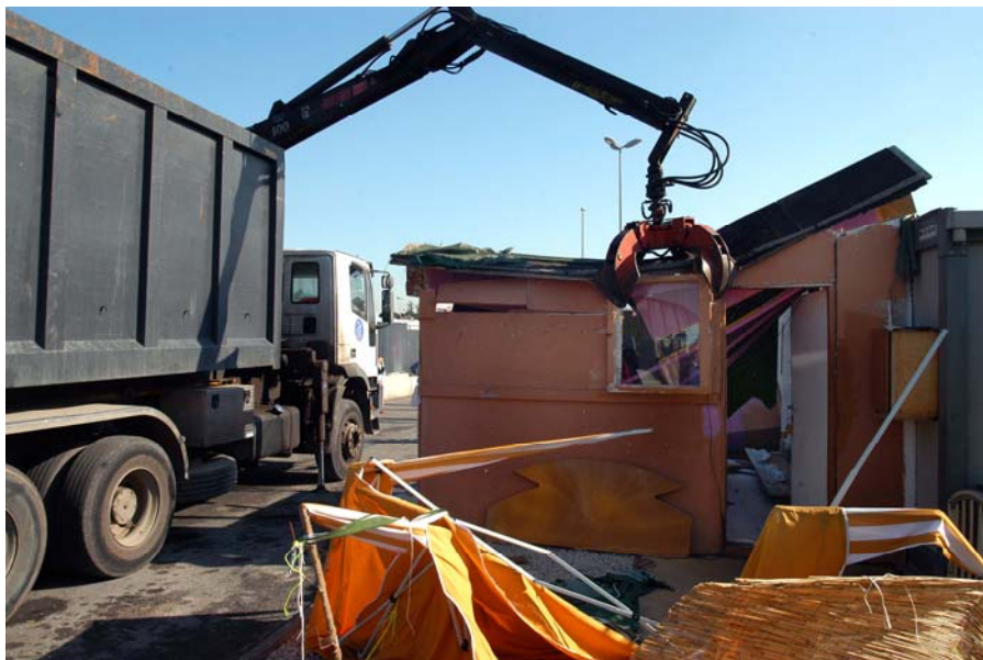
Demolition of a shack, via Gordiani camp, Rome, November 2007
